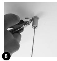
Cut the Suspension Wire to the desired Wire length.
